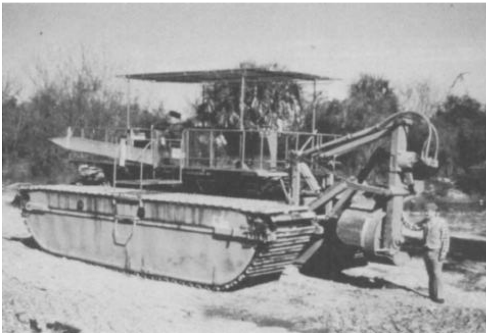
Figure 5-16. Track-mounted rotary trencher used in mosquito control activities
